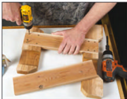
Set the vertical slats securely into their notches with weatherproof glue and exterior-grade screws for outdoor durability.
