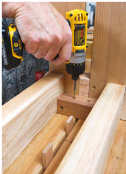
Upend the bench and table frames onto the 2x6 top boards, and drive 3" screws through the cleats to hold them in place.
